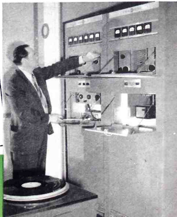
Dwelle S. Hoag, Chief Engineer of W47A, takes readings on the 1-kw FM transmitter
