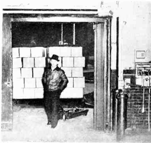
Photoelectric door opener saves many times its cost of installation
